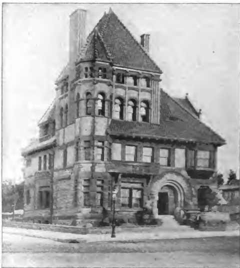
RIVERBIDE DRIVE, CORNER OF 108TH STREET. RESIDENCE OF SAMUEL G. BAYNE.
